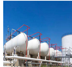
Fuel oil pumps
