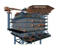
PH accommodation Platform four legs, 22 m water depth, UK North Sea. Total weight 5000 tons. Detail Design of Jacket, Deck, Helideck and Bridge
