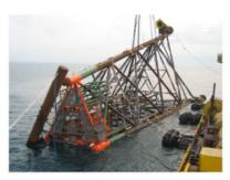
Offshore Congo Two Drilling and Production Platforms installed in 80 m water depth.
