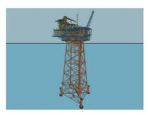
Marlin Drilling and Production Platform in 110 m water depth. Four leg Jacket, Deck and Living Quarter. Platform total weight 8.500 tons
