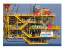
Well Head Platform four legs in water depth of 28.5 m in Mediterranean Sea installed on a pre-existing submarine well template
