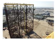
Hasbah and Arabiyah Offshore Fields N\* 2 Platforms 8 legs in 45.3m and 51.4m water depth. Weight of each platform 8.000 tons
