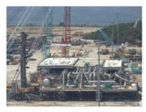
Iraq Crude Oil Export Expansion Project (ICOOEP) CMMP Platform 8 leg in Persian Gulf water depth of 27.5 m Topside installed by Float-over Mating
